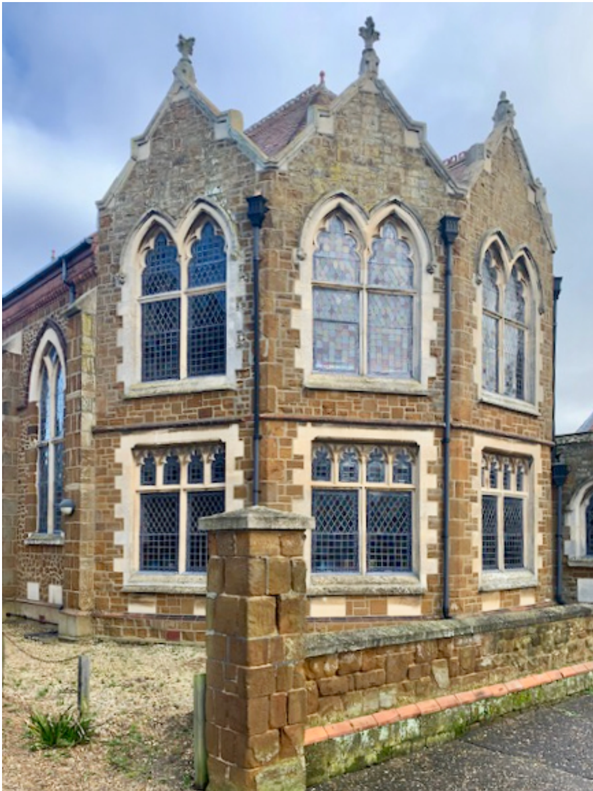
The Wesleyan Chapel was opened alongside the 'tin hut' on 15 June 1896, on what was to become the junction of the High Road and Austin Street. The carrstone building was constructed by William Jarvis of King's Lynn, for £1,540.
